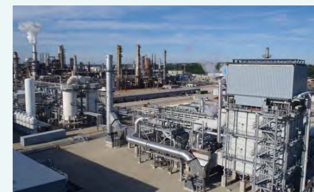
Existing HyCO plant
