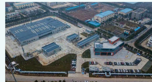
Electronic materials gases production plant in Yangzhou, China
